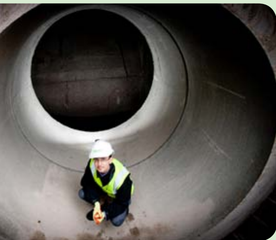
Top - Screening chamber that will house 3 powered screens.
